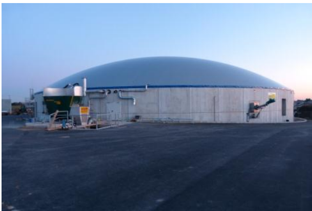
Biogas plant at Pirmasens-Winzeln Energy Park
