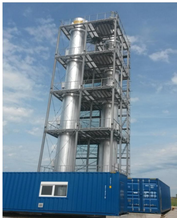
PFI engineering lab scale plant for methanation and power-to-gas pilot plant built at Pirmasens Energy Park
